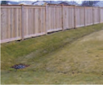
Typical backyard swale with a drain.
